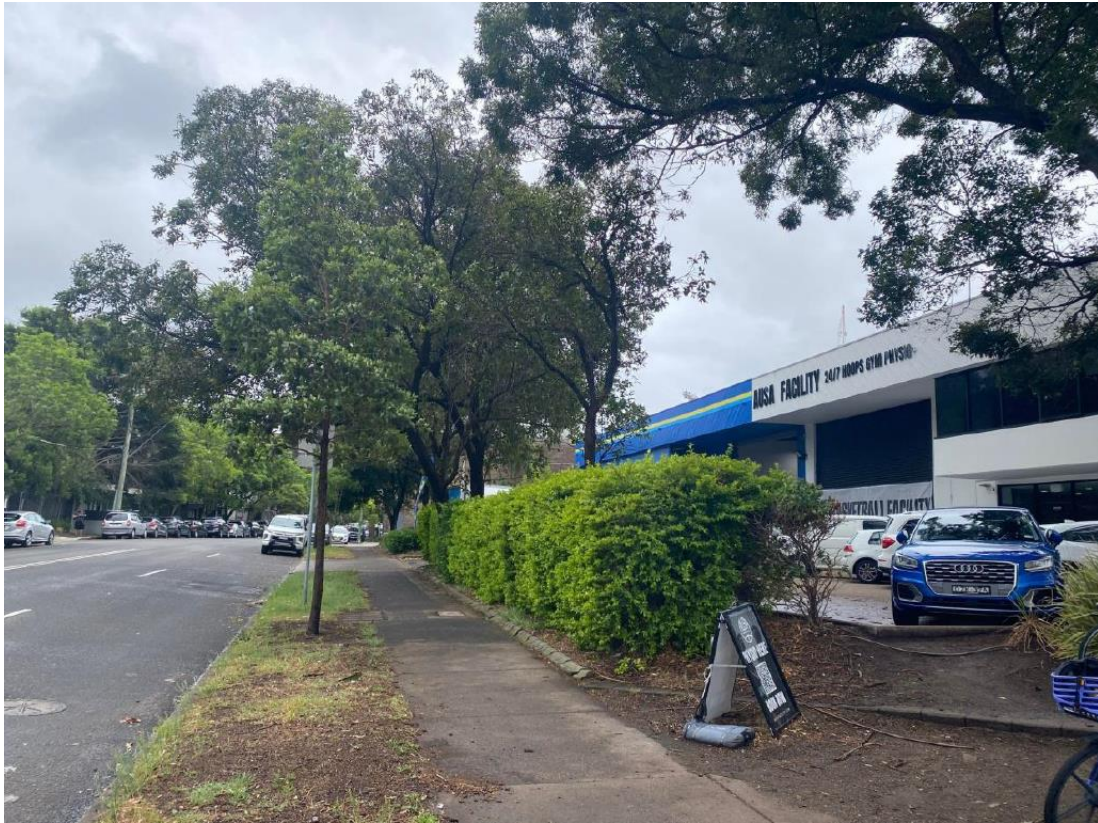
Figure 3: Site viewed from Wyndham Street looking north
